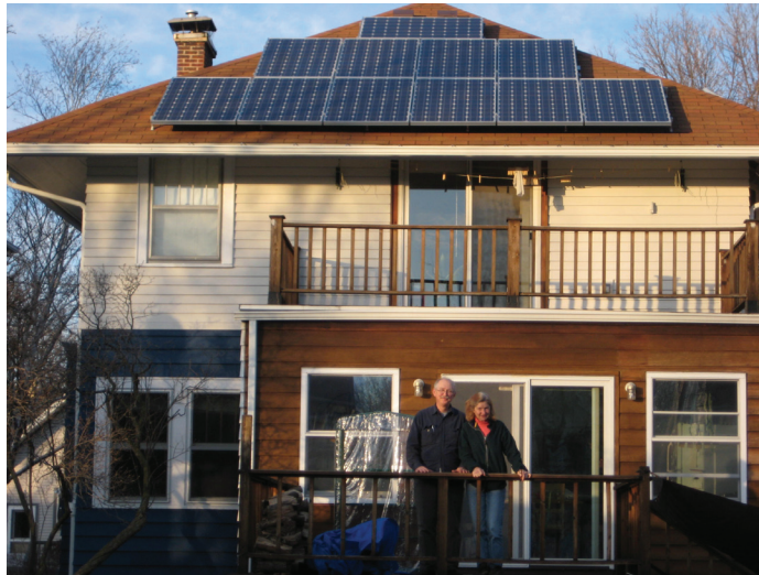
A view of the solar panels on the rear roof; the rest of the panels are on the southern side of the house.
